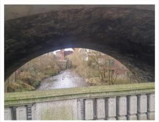
**The solution:** Prior to the concrete repair programme, existing coatings were first removed via scraping and washing, in order to provide a sufficient key for repairs. A hammer test was undertaken to the shotcrete render covering the arch intrados before a cementitious repair
